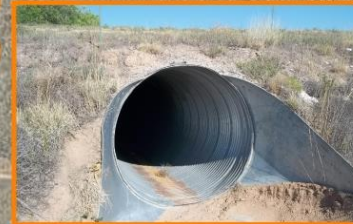
Clean Existing Culverts
