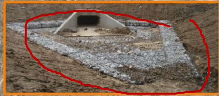
Downstream Riprap Placement
