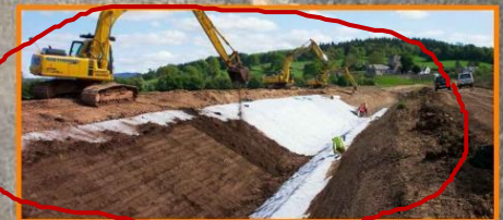
Sediment Basin and Channel Installation
